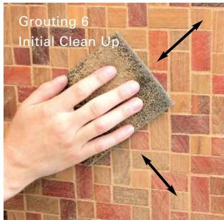
Begin initial cleaning when the grout film just starts to dry on the surface of the tiles. Depending on temperature, humidity and air flow at the installation site, this could be between 5 and 10 minutes. Using one of the provided scotchbrite pads, dampen -- **NOT WET**-- the pad and scrub the residue on the tile surface working in a diagonal motion to the grout joints. This will create a uniform slurry of grout residue on the surface of the tiles.
