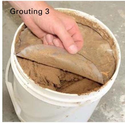
The area to be grouted before starting initial clean up will depend on ambient temperature and humidity conditions and air flow at the installation site. **Start by grouting a few square feet at a time to check grout drying time before grouting a large area.**
