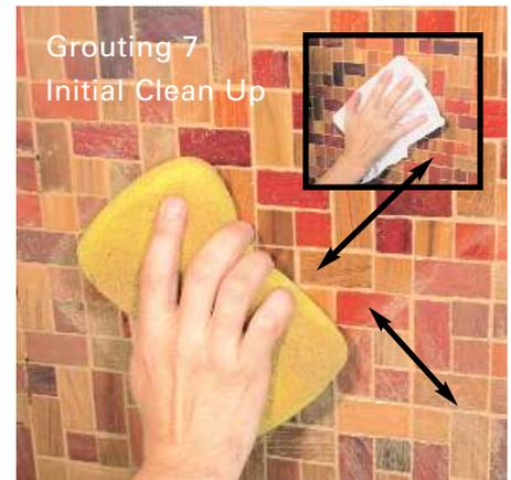
Using a new, clean, slightly damp -- **NOT WET**-- sponge, clean off the surface film by working in a diagonal motion to the grout joints. Be careful not to remove excess grout from the grout joints. Rinse the sponge frequently using 2 buckets of water: one for rinsing out the heavy residue, the next for rinsing the sponge with clean water.
