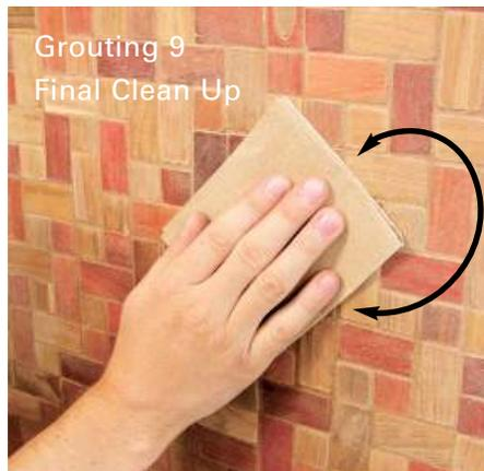
Using the provided 220 grit sandpaper lightly sand the surface of the tiles using a random circular motion. For 1x2 inch mosaic patterns and liners sanding in the direction of the grain is recommended.
