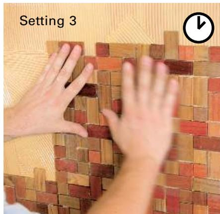
When setting tiles in a vertical application, comb an area of a few square feet at a time as instructed above and then let the adhesive set until the adhesive no longer "sags" before applying the tile sheets.
