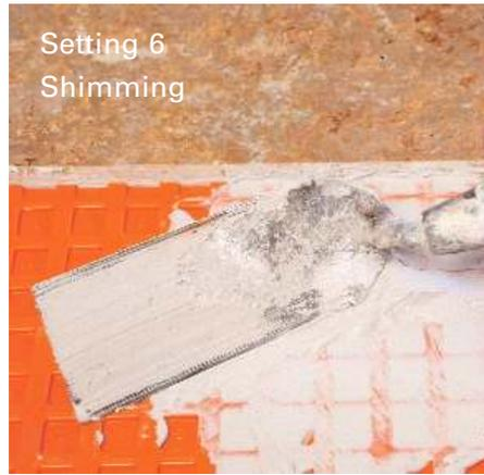
When installing Fortis Arbor tiles next to  $\frac{3}{8}$  inch stone or tile you can "shim" up the wood tiles with Schluter Ditra Universal Underlayment. Once the underlayment is applied you must fill the "waffle" side of the underlayment with thinset mortar and let it thoroughly dry. At that point you can set the wood mosaics tiles on the underlayment as previously described.
