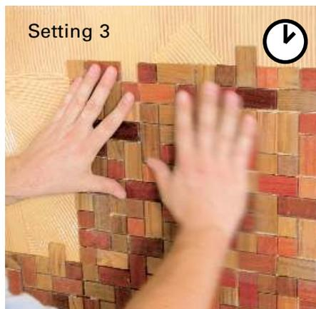
When setting tiles in a vertical application, comb an area of a few square feet at a time as instructed above and then let the adhesive set until the adhesive no longer "sags" before applying the tile sheets.
