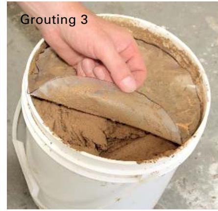
The area to be grouted before starting initial clean up will depend on ambient temperature and humidity conditions and air flow at the installation site. **Start by grouting a few square feet at a time to check grout drying time before grouting a large area.**
