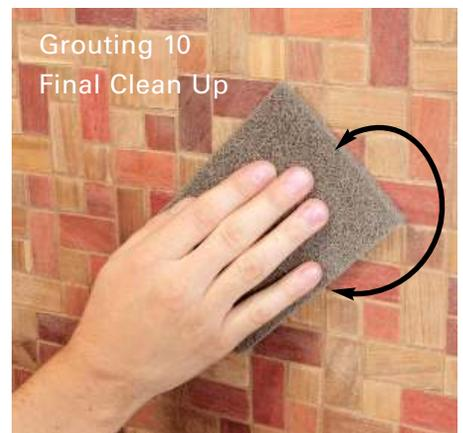
Using the 2nd provided scotchbrite pad lightly buff the surface of the tiles using a random circular motion.
