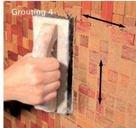
Spread grout over the face of the tiles using a rubber grout float. Holding the float at a 45° angle to the face of the tile, work in a parallel motion to the grout lines to ensure completely filling the joints.
