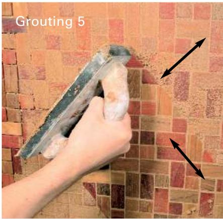
Remove excess grout by holding the float at a 90° angle to the face of the tile and working diagonally across the grout lines.
