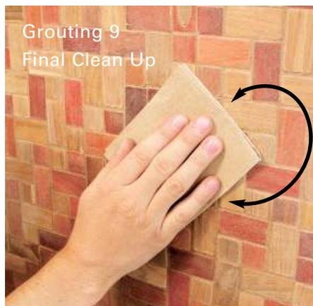
Using the provided 220 grit sandpaper lightly sand the surface of the tiles using a random circular motion. For 1x2 inch mosaic patterns and liners sanding in the direction of the grain is recommended.
