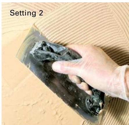
Use a  $1/8 \times 3/32 \times 3/32$  inch U notched trowel to apply the adhesive. Apply a thin coat of adhesive with the flat side of the trowel to ensure a good mechanical bond. Comb adhesive with U notched trowel listed above. Periodically check for at least 80% adhesive coverage on the bottom of the tiles.
